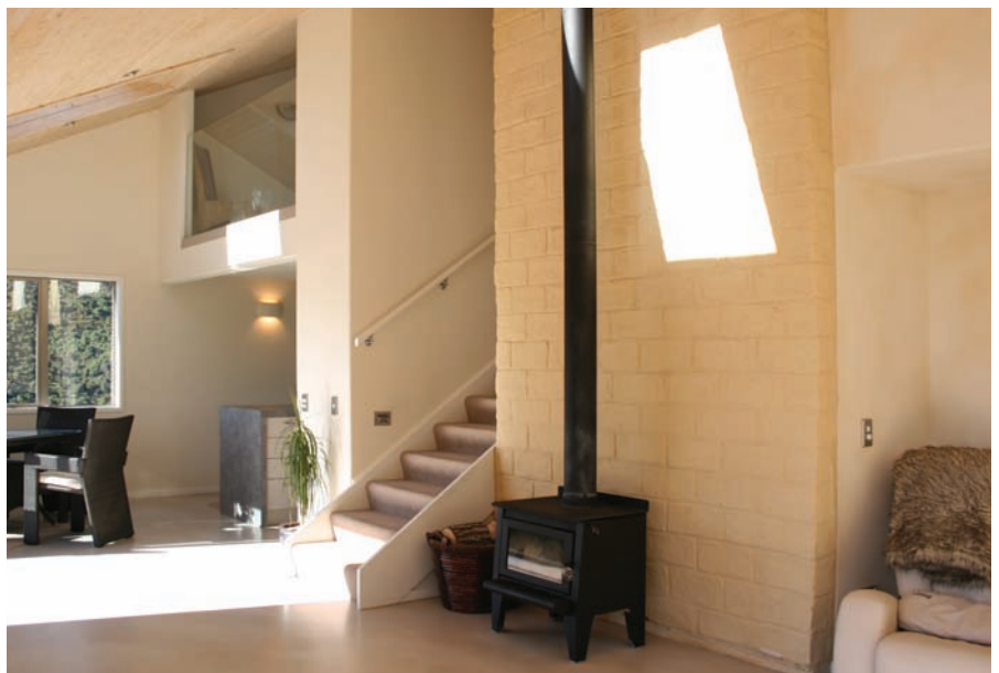
Locally sourced adobe blocks and concrete floors are used as a thermal mass. A small efficient wood burner complements this passive heating.
